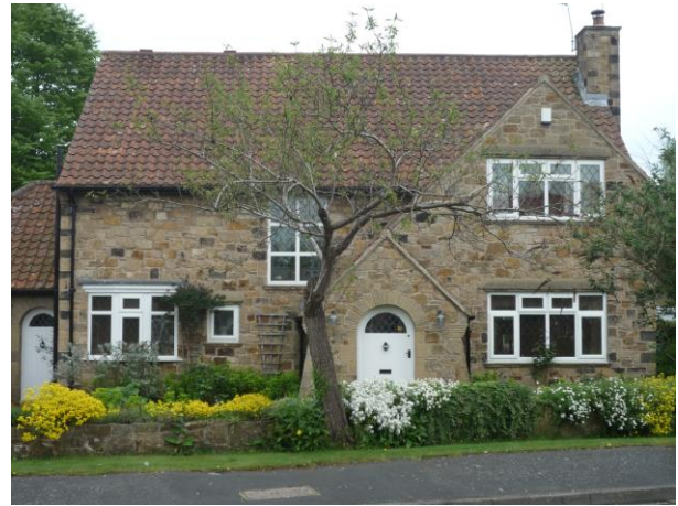
Photo 14.5 Porch with Roman Arch
