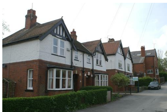
Photo 14.2 Forward facing gables
