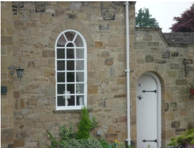
Photo 14.4 round-headed window and door
