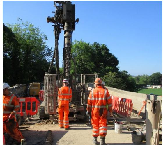
*One of the 13 piles being drilled through the south pier.*
