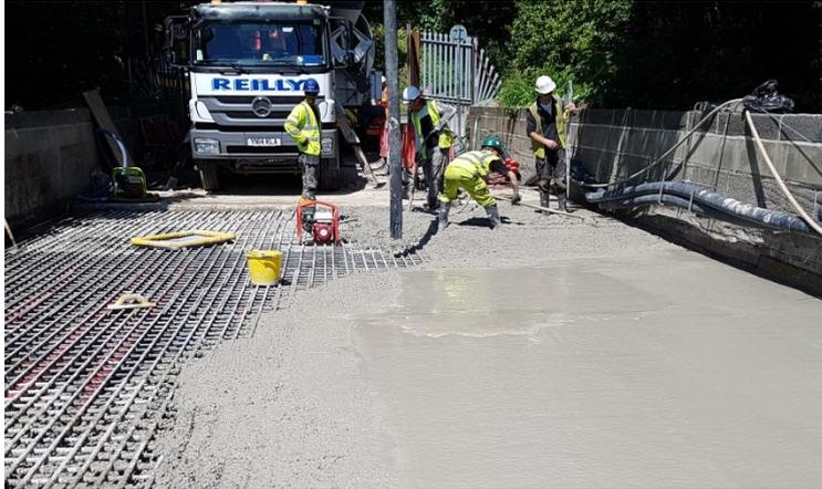
*Placing reinforced concrete to the north arch slab.*
